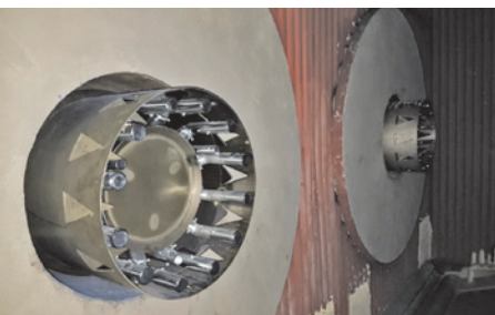
Obr. 8 hořáková Low-Nox hlava, hořák Elco RPD 70 G-EU2
