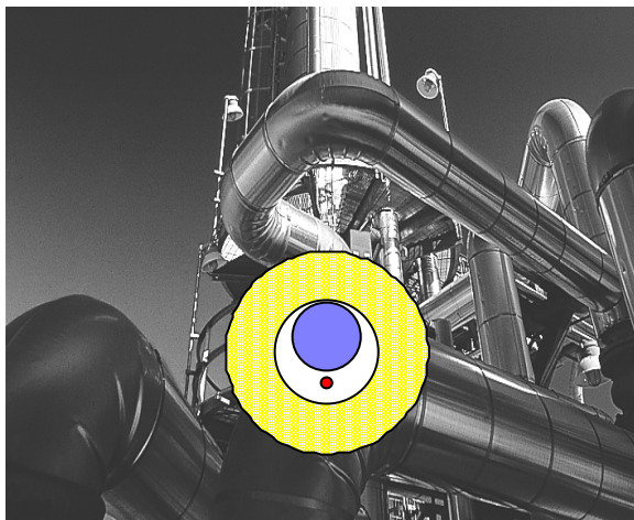
Due to the influences of the specific installation no responsibility is accepted for the correctness of this calculation.
